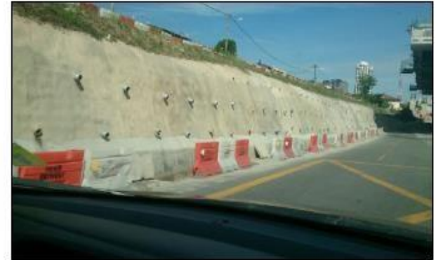
Photo 24: Duta - Ulu Kelang Expressway (Duke) Phase 2: Soil Nailing, Guniting And Horizontal Drain Work At Jalan Lang Hitam
